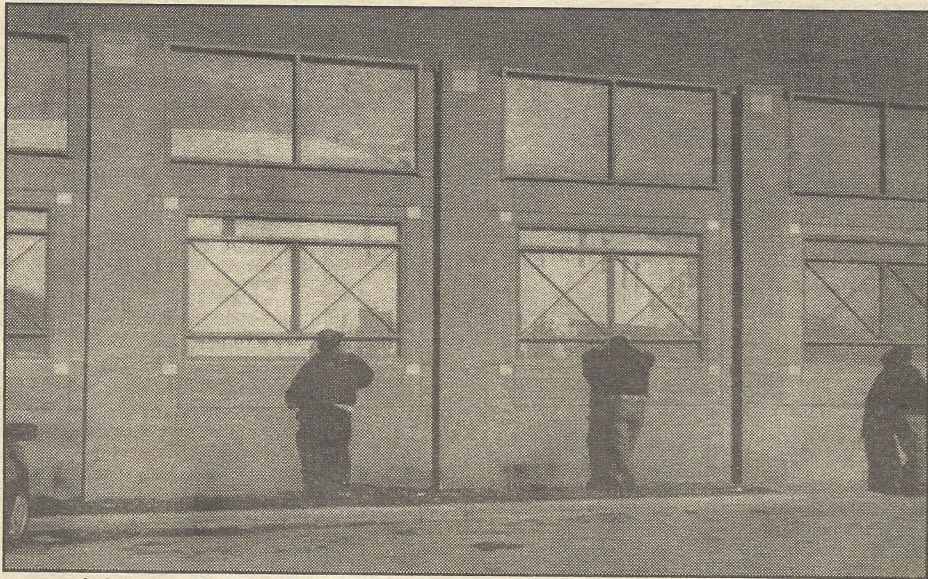
Men peak through new, "friendly-looking," 14-ft border fence from Nogales, Mexico into Nogales, Arizona.
